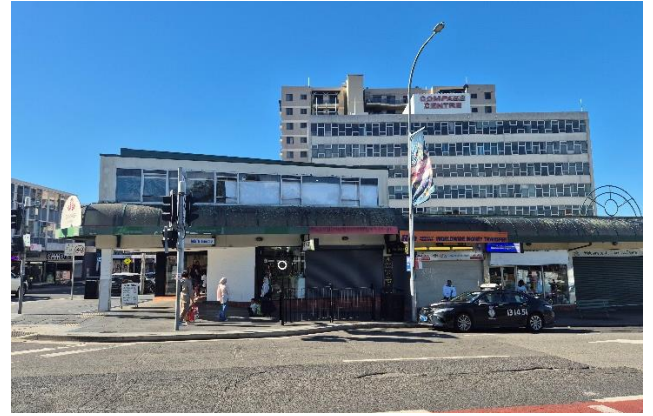
Existing development as viewed from Swane Reserve to the south
