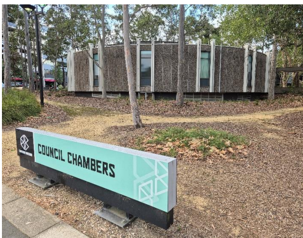
Bankstown Council Chambers to the north-west of the site
