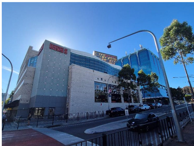
HOYTS Bankstown to the north-east of the site and the Bankstown Civic Tower to the right of the image
