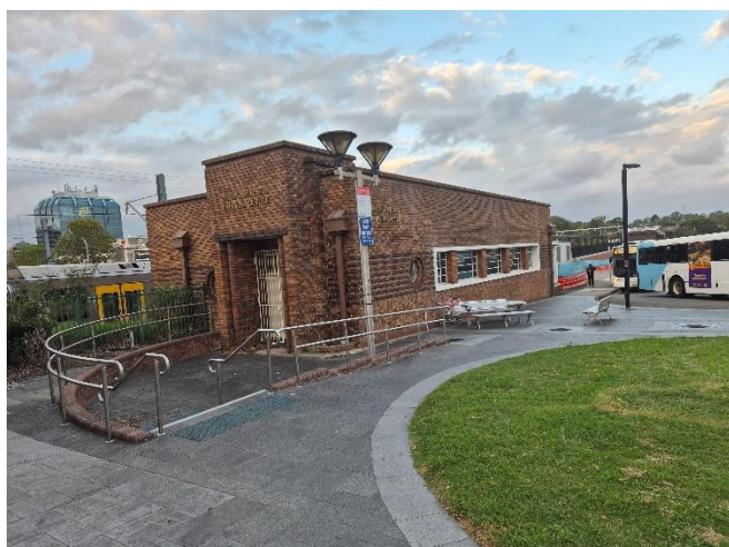
Heritage significant former Bankstown Parcels Post Office which is to be demolished to accommodate the future Bankstown metro station
