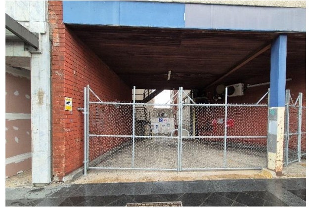
Car park access to the west of the site from Fetherstone Street
