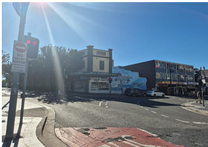
Fine grain retail, office and business uses to the west of the site along Fetherstone Street
